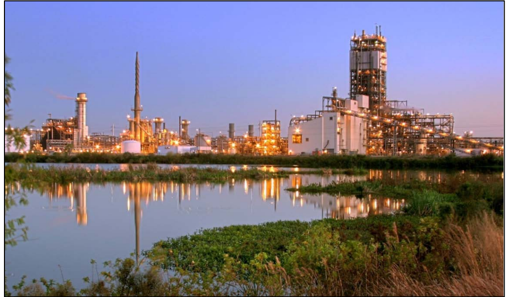
Polk Power Station, Unit
